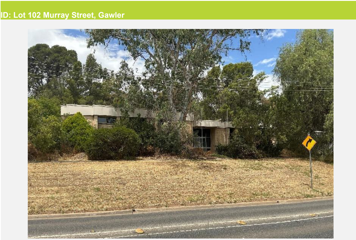
Figure 1, Street View of Lot 102 Murray Street, Gawler
