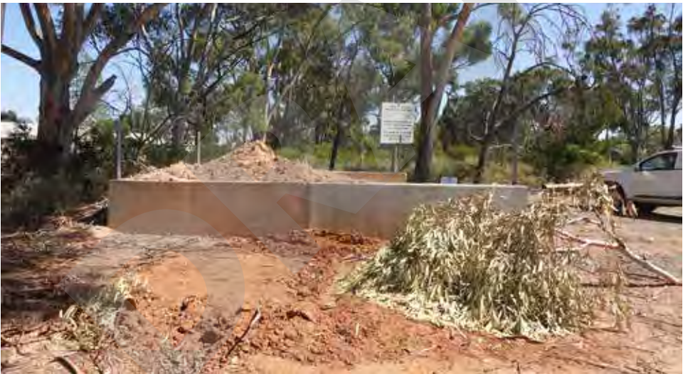
▲▲ Figure 2.2 Main north-south roadway looking north towards centre of circle.
