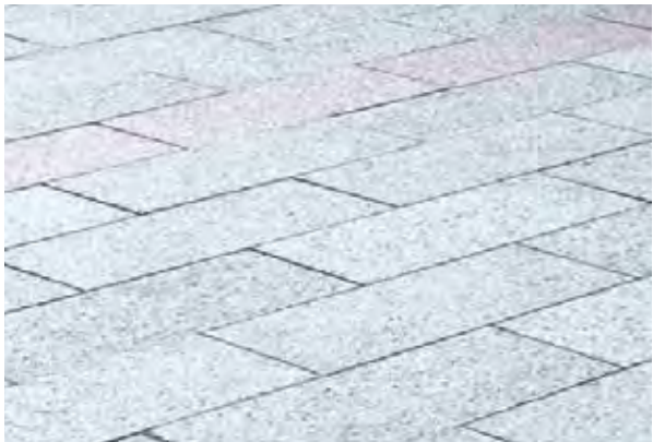
Granite Pavers Colour: Adelaide Black Finish: Light washback finish in compliance with P5 slip rating Application: Entry Node/ Around Columbarium
