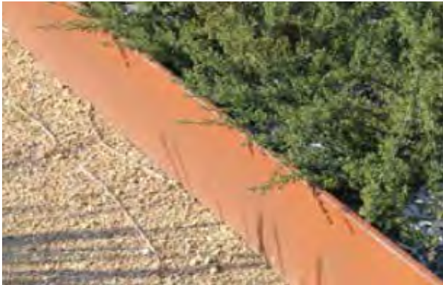
Steel Edging Colour/ Finish: Rusted finish ; HDG Application: Garden Edging in Focal Nodes ie. columbarium
